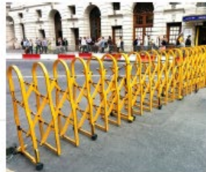
Temporary scissor barriers deployed to close footpath when vehicles access site. Footpath reopened between vehicle movements.
