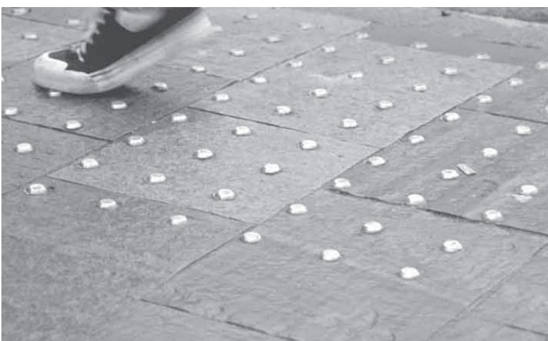
Steel studs and strips applied to warn of hazards (such as steps)
